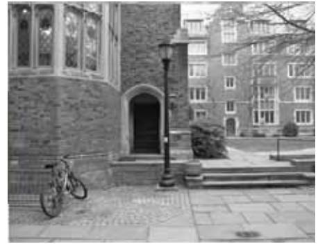
Existing conditions, courtyard entry.
